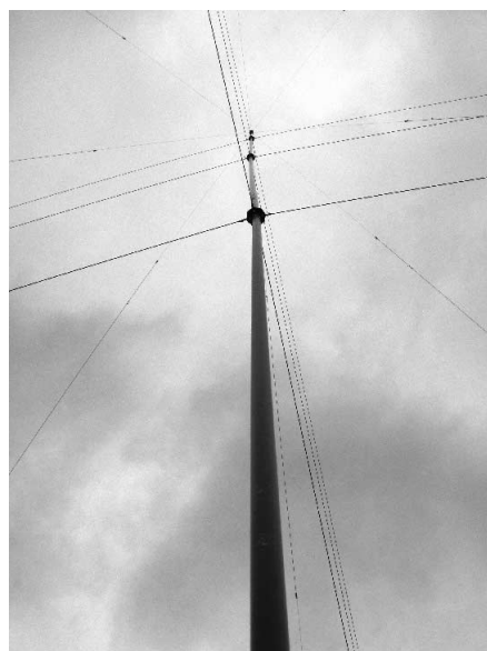
Figure 5 — Looking up the 82 foot mast to the top loading at M8M (viewed from the side it looks straight!) [G3LNP photo]
